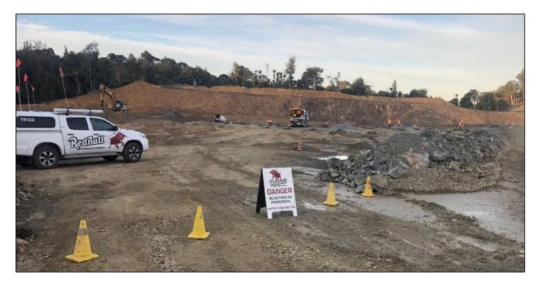
A risk assessment should be completed for each blast, identifying the hazards and controls at each stage, including the extent of the blast exclusion zone during the firing sequence. Any risk assessment and subsequent hazard controls should be agreed to and approved by all the relevant parties involved in the blasting process before blasting.
